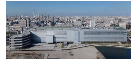
Next-Generation Large-Scale Distribution Center: X FRONTIER
